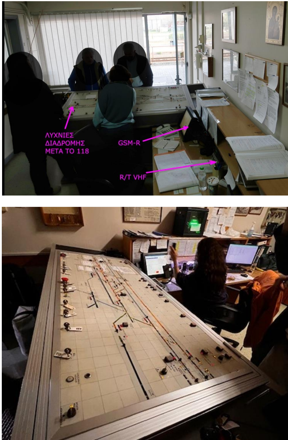
Figure 41. Positions of station masters when facing the control panel (above) and when communicating (below) in Larissa station.
