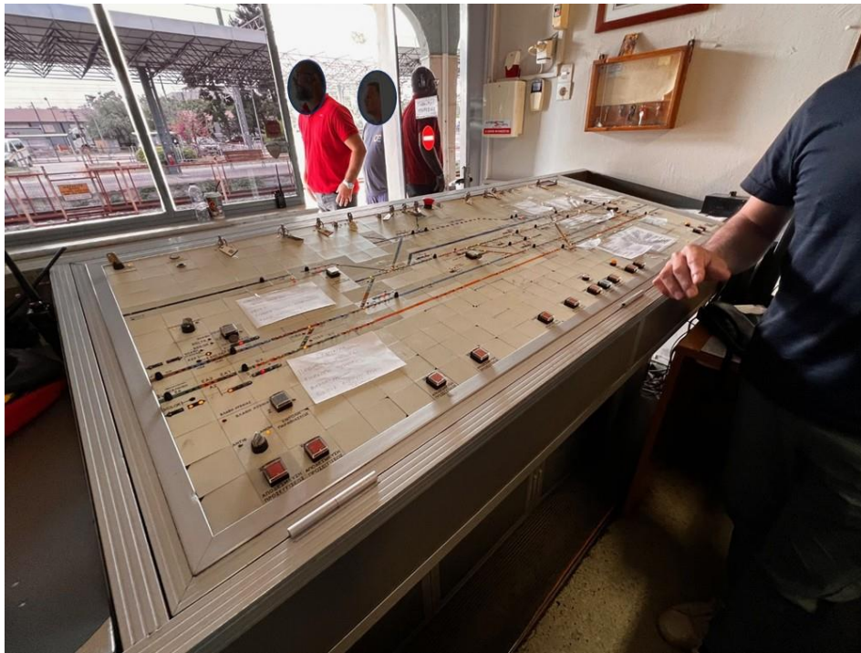
Figure 37. The control panel at Larissa Station
